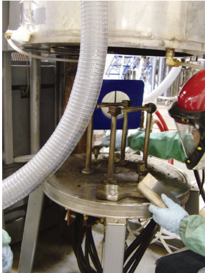
Figure 20. Local exhaust ventilation and PPE used during reactor cleanout.
