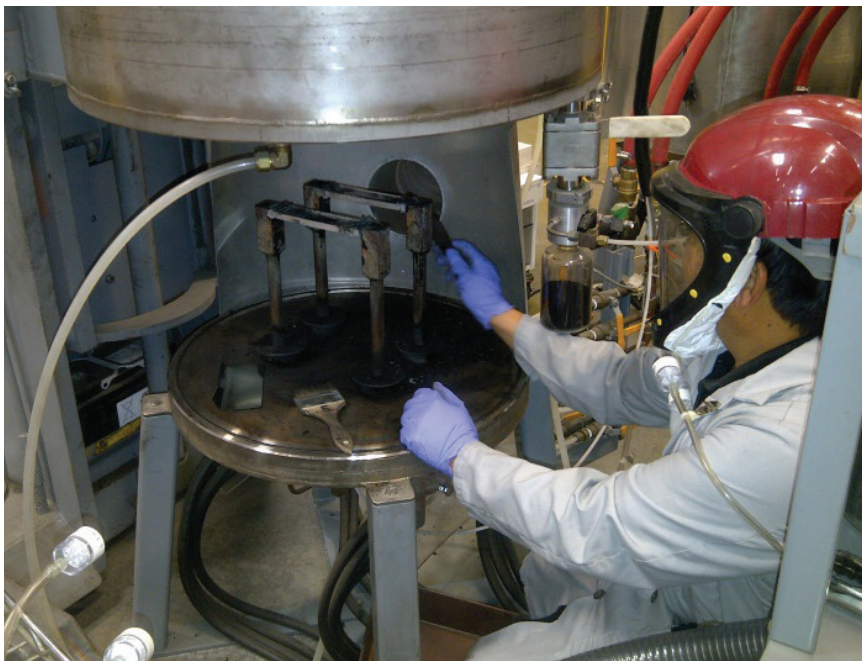
Metal oxide reactor cleanout
