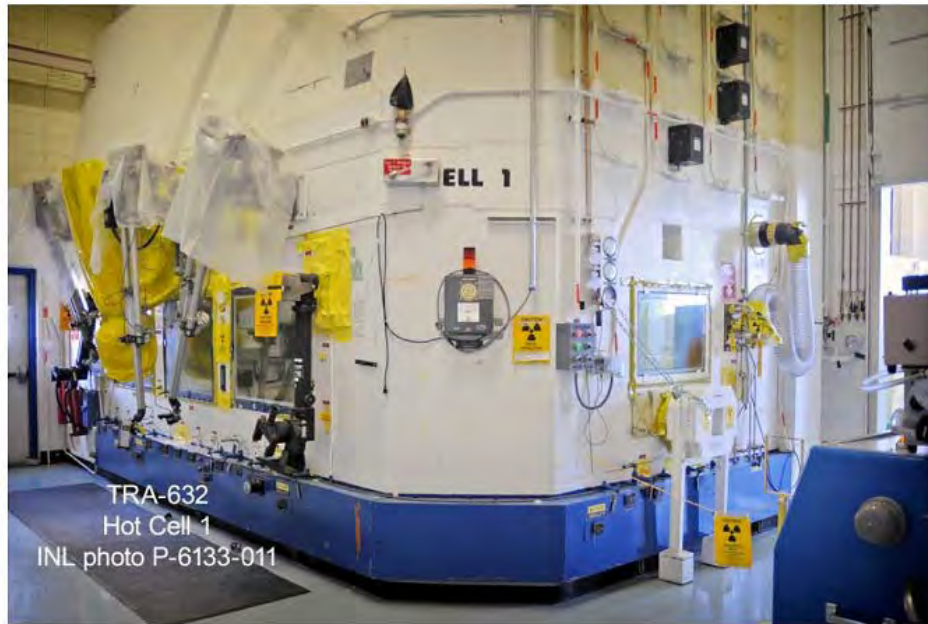
Figure 5-14: TRA Hot Cell #1
