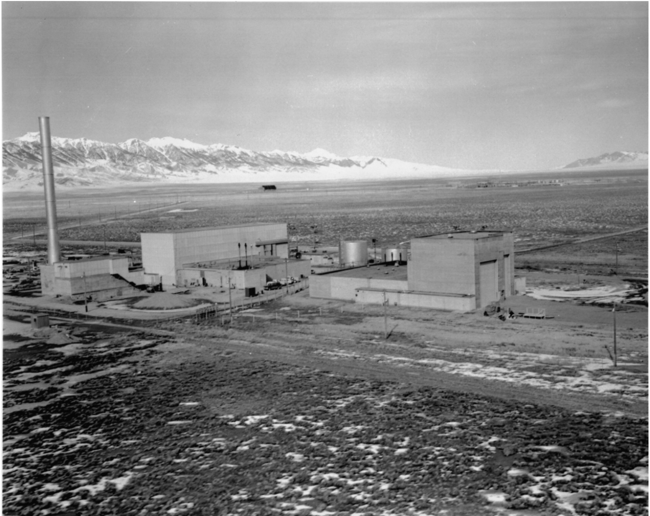
Figure 5-38: Photograph of the LPTF Area (looking northwest)
