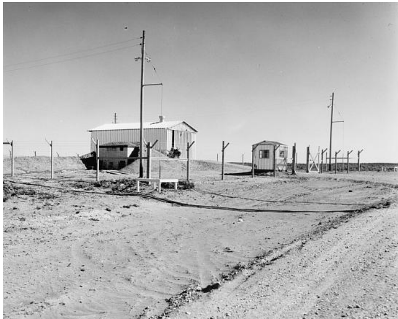
Figure 5-54: The SPERT-I Facility
