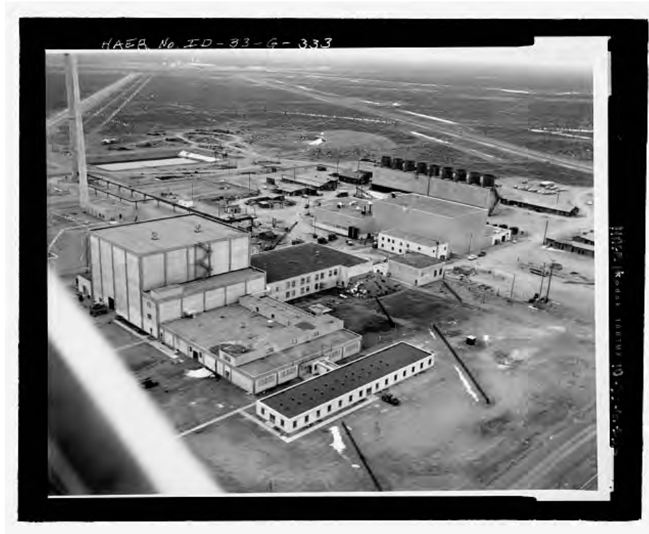
Figure 5-5: Test Reactor Area (TRA) Complex, 1956
