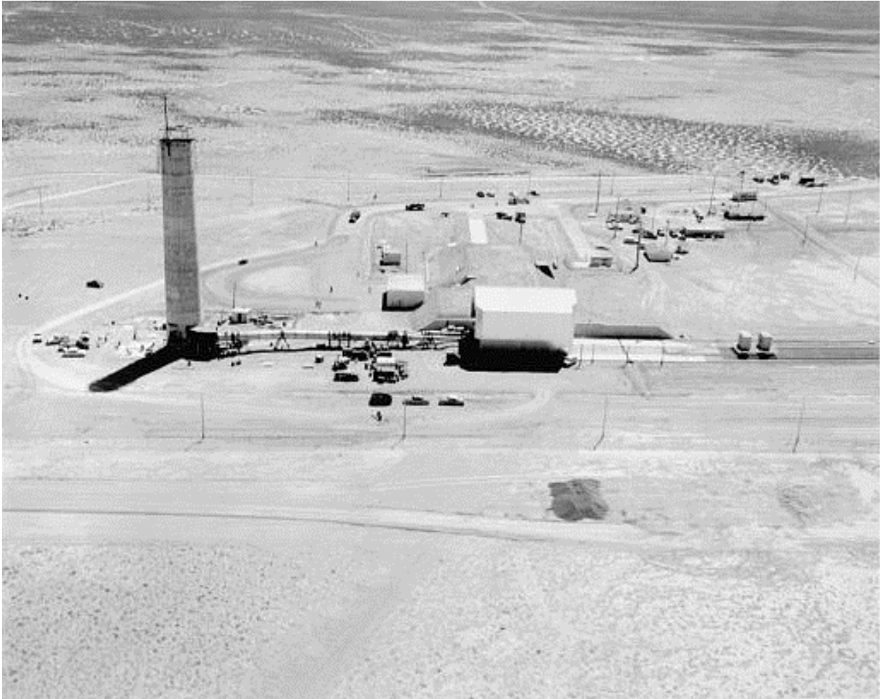
Figure 5-34: Aerial Photograph of the IET Facility (facing east)
